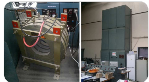
Load inductor (100kg), load resistor (wall closet)
